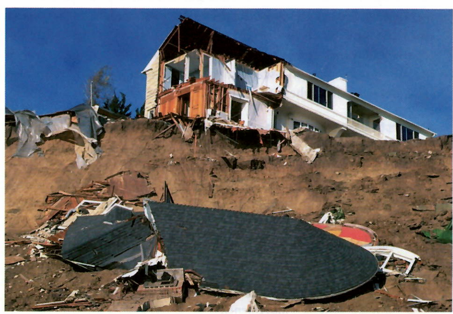
Figure 19 Landslide This home in Pacific Palisades, California, was destroyed by a landslide triggered by the January 1994 Northridge earthquake.
