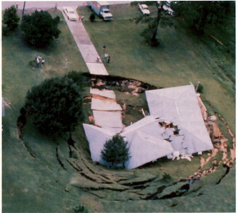
Figure 24 This small sinkhole formed suddenly in 1991 when the roof of a cavern collapsed. It destroyed this home in Frostproof, Florida.
