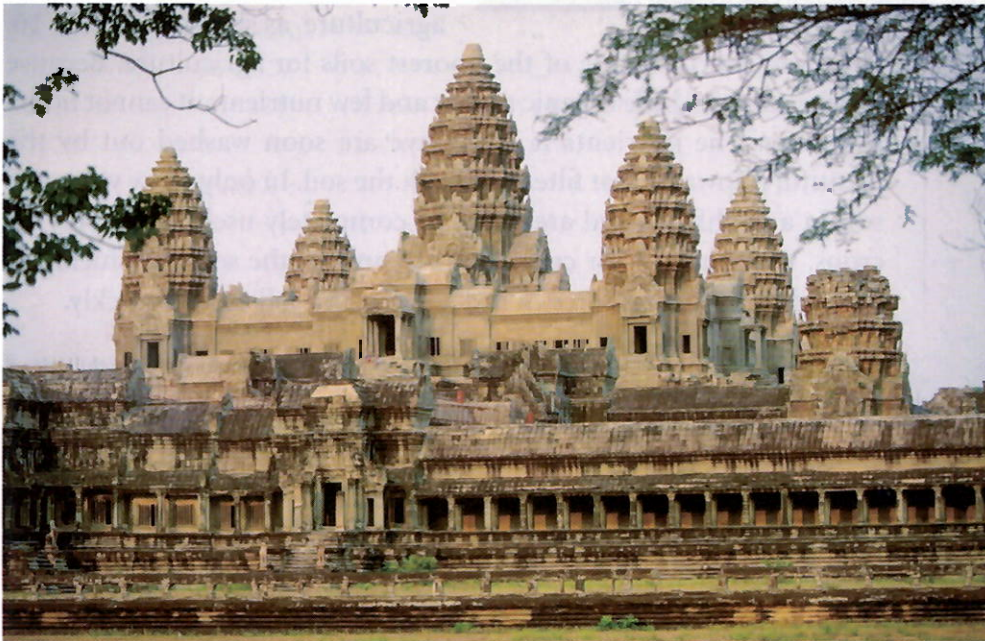
Figure 15 The Temple at Angkor Wat, Cambodia This temple was constructed of laterite bricks between 1113 and 1150.
