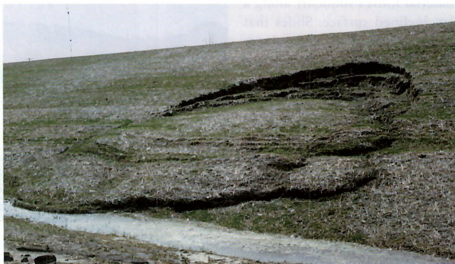
Figure 23 Earthflow This small, tongue-shaped mass movement occurred on a newly formed slope along a recently built highway.
