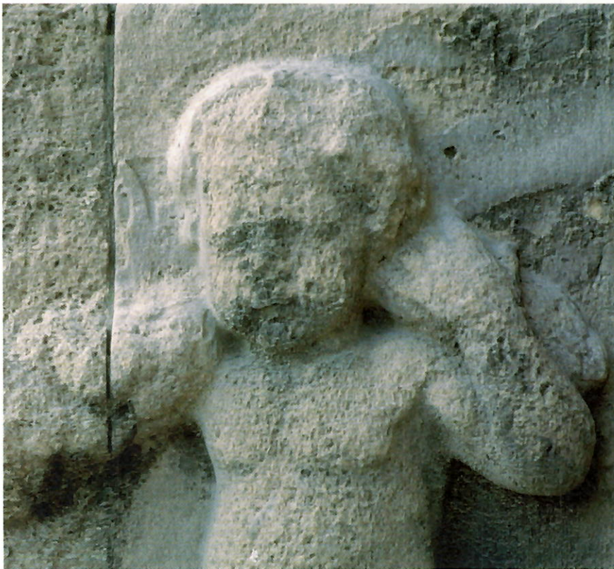
Figure 7 One Effect of Acid Precipitation Acid precipitation contributed to the chemical weathering of this stone building facade in Leipzig, Germany.
