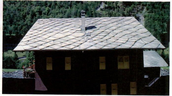
Figure 4 The roof on this house is made of slate. Slate is a metamorphic rock that forms from the sedimentary rock shale. Explaining How can shale become slate?
