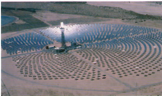
Figure 9 Solar One is a solar installation used to generate electricity in the Mojave Desert near Barstow, California.
