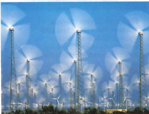
Figure 12 These wind turbines are operating near Palm Springs, California.
