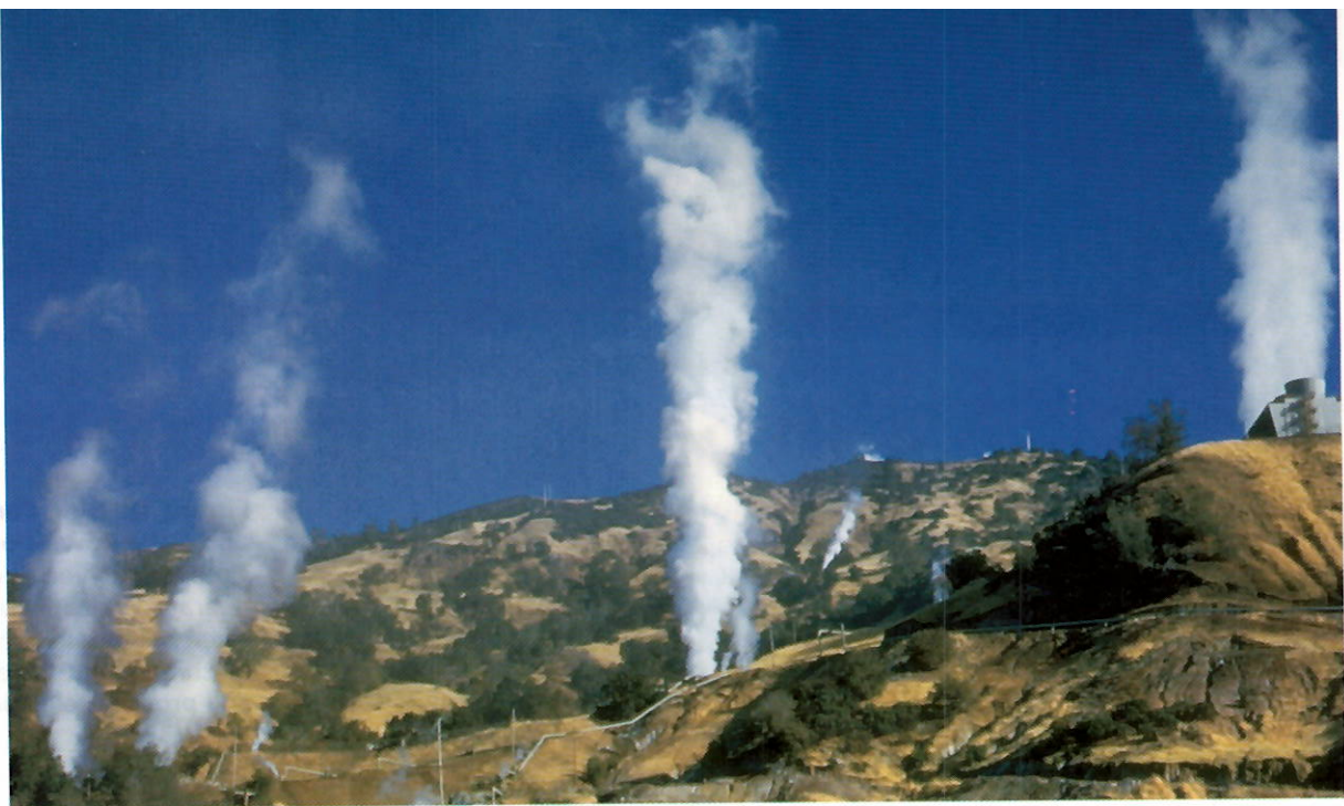
Figure 14 The Geysers is the world's largest electricity-generating geothermal facility. Most of the steam wells are about 3,000 meters deep.
