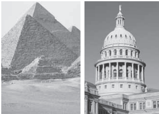
The ancient Egyptians used a rock called limestone to build the pyramids at Giza (left-hand figure). The Texas state capitol building in Austin is constructed of a rock called granite (right-hand figure).
