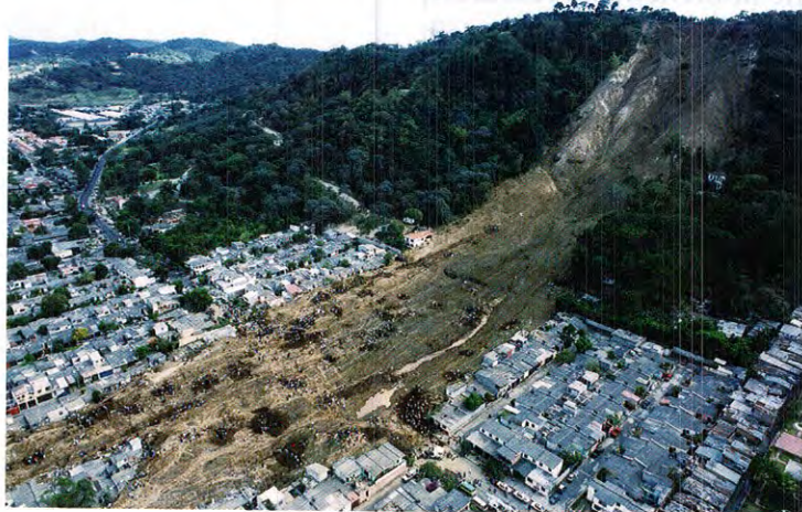
Figure 22 The damage here was caused by a landslide that was triggered by an earthquake.
