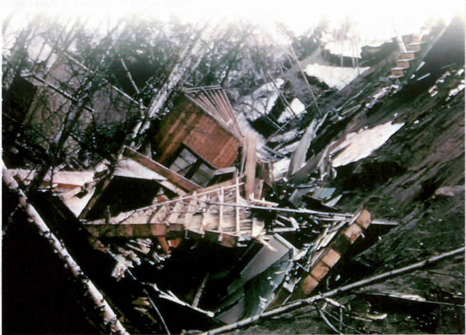
Figure 12 This landslide caused by the 1964 Alaskan earthquake destroyed many homes. More than 200 acres of land slid toward the ocean.
