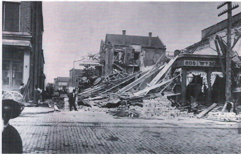
Damage to Charleston, South Carolina, caused by the August 31, 1886 earthquake.
