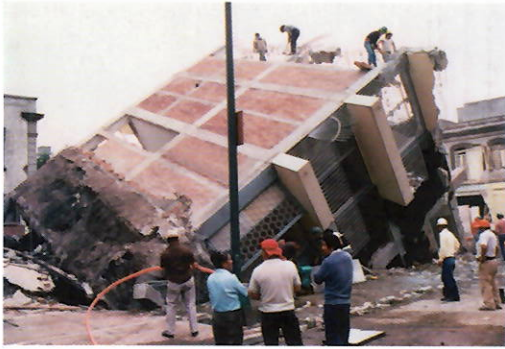
Figure 13 Effects of Subsidence Due to Liquefaction This tilted building rests on unconsolidated sediment that imitated quicksand during the 1985 earthquake in Mexico.
