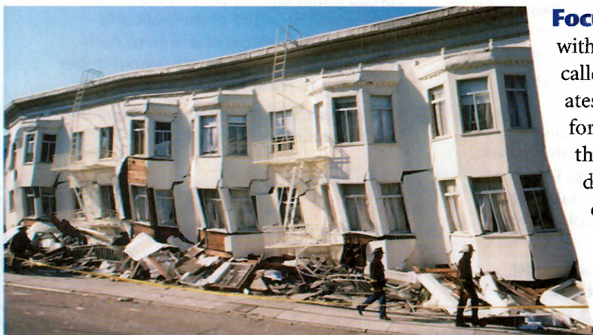
Figure 1 This damage occurred in San Francisco's Marina District from the 1989 Loma Prieta earthquake.
